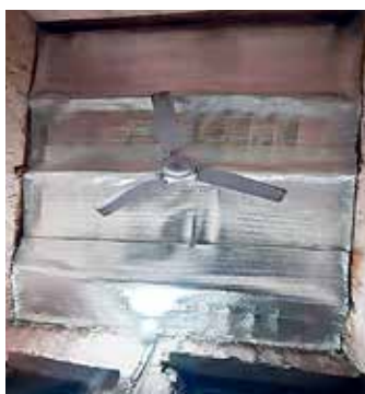
FIGURE 8: Alufoil layering under roof
